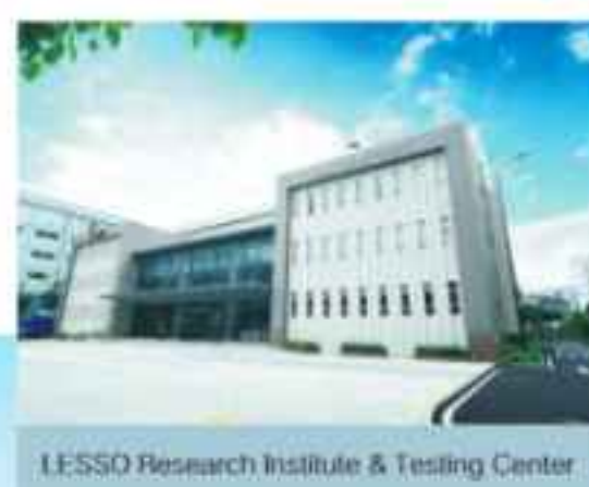
LESSO Research Institute & Testing Center
